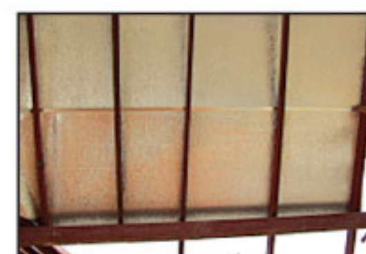
Step 7 View from roof underneath.
