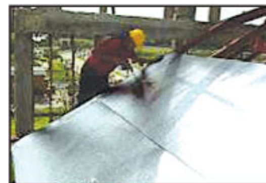
Step 3 Using self-tapping screw for light weight trusses or stapler for timber trusses to secure CoolMax™.
