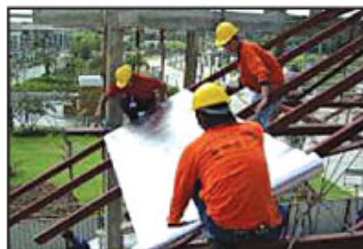
Step 2 Starting from trusses edge, lay CoolMax™ across the purlins.
