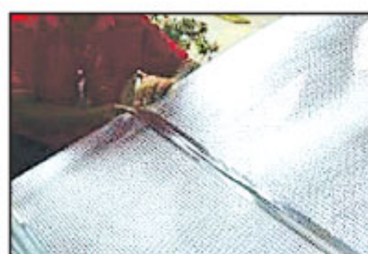
Step 4 Make sure overlapping shall be at least 50mm and stick with PP all weather tape which is heavy duty self extinguished tape.
